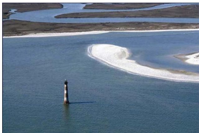
Fig. 2— Morris island light house on land during W.W. II, in Southern California, USA, now inside Sea (Source: http://www.savethelight.org/gallery200705to200706.html#stayhere )
