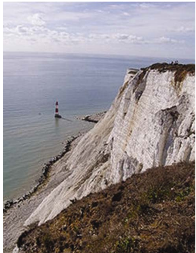
Fig. 5(a) — Cliff erosion in UK (Source: http://en.wikipedia.org/wiki/Beachy_Head ).
