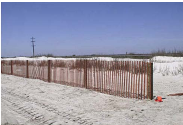
Fig. 15— Sand fencing on an US beach (Source: http://www.gulfmex.org/crp/7004/fence.jpg ).
