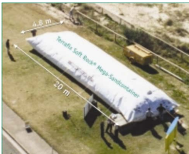
Fig. 13— Terraflx soft rock geotextile sand container (Source: http://www.globalsynthetics.com.au/files/introduction_coastal.pdf ).
