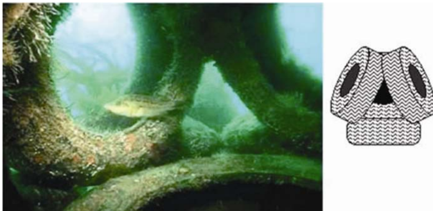
Fig. 9— Tetrahedral design of tyres used in artificial reef in Poole Bay, Dorset, UK (Courtesy of Dr. K.J. Collins; Source: HR Wallingford, UK).
