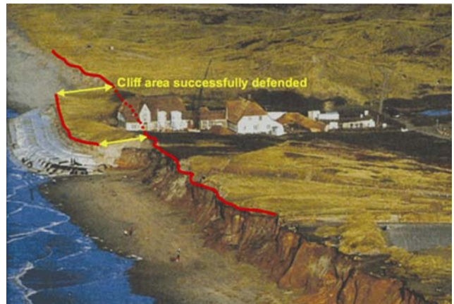
Fig. 14(b) — Defended cliff area with geotextile sand cushions on the Island of Sylt, Germany (Source: http://www.coastalmanagement.com.au/papers/GeoEng00.pdf ).
