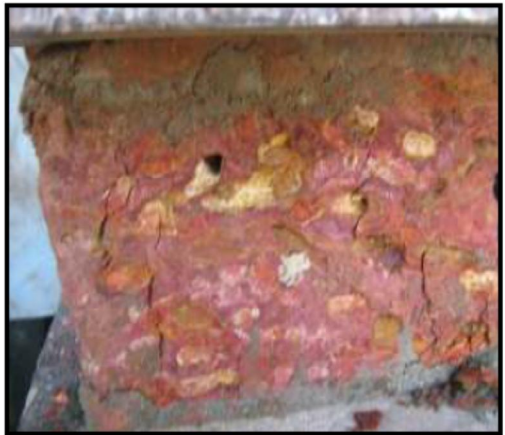
Figure 2: Failure Pattern in Laterite under Compression
