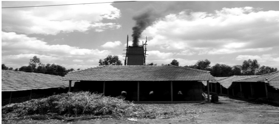
Figure 2 Kilns for burning bricks (see online version for colours)
