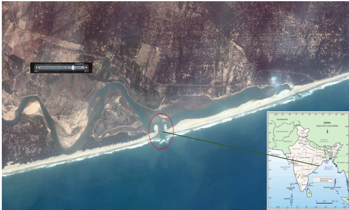
Figure 4.2(b) Study area [Google Earth image as on 14-01-2014 (i.e. after Phailin cyclone)]
