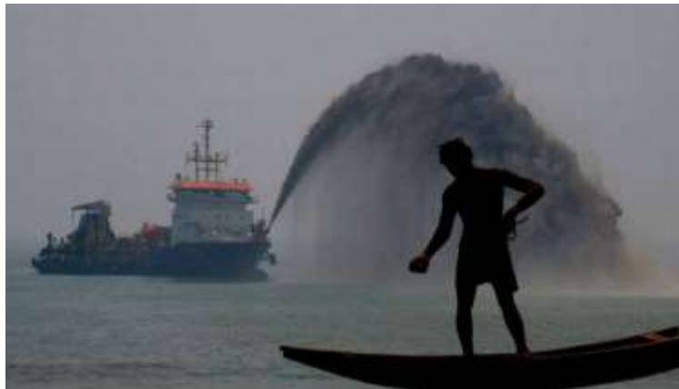
Plate 2.2 Dredge-21, a vessel of the Dredging Corporation of India pumps sand water as part of beach nourishment (Source: The Hindu, Photo Credit: K R Deepak)
