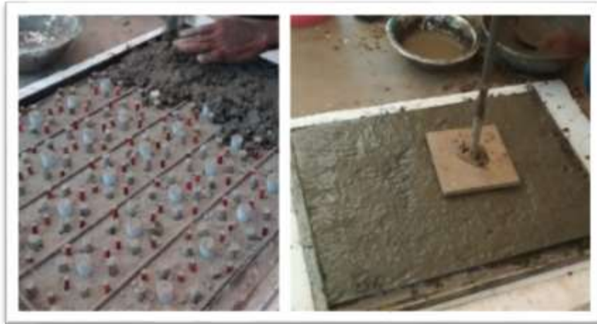
Plate 3.5 Preparation of the base slab
