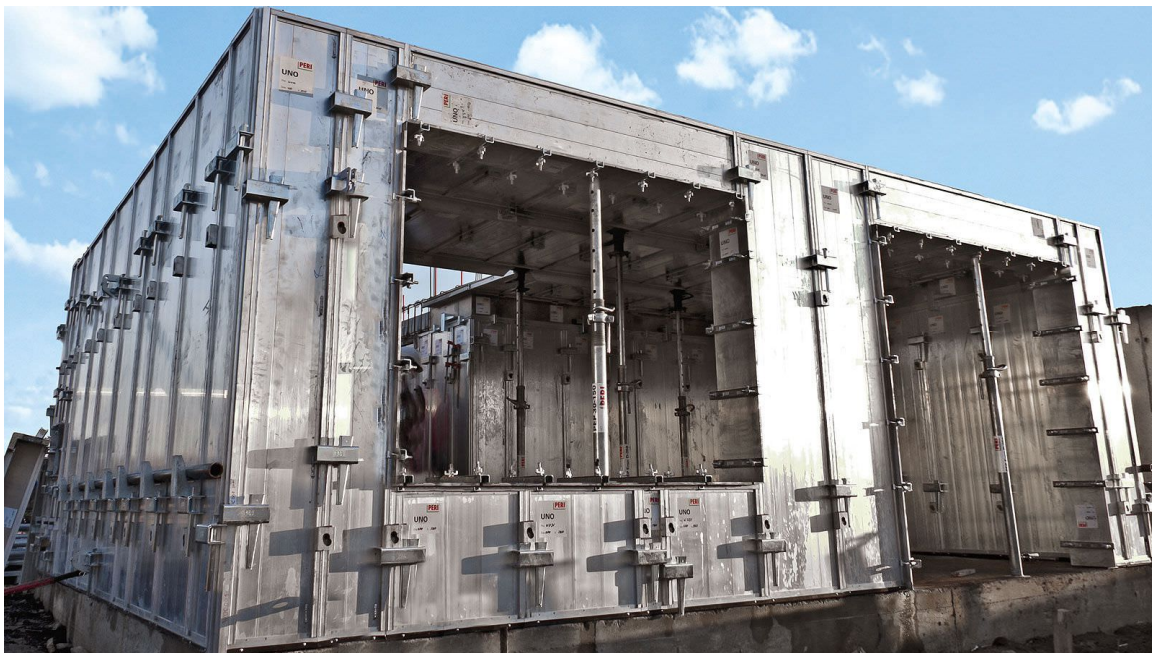
Fig 4.9 Aluminum panel monolithic construction (Source: Directindustry-Monolithic formwork)
