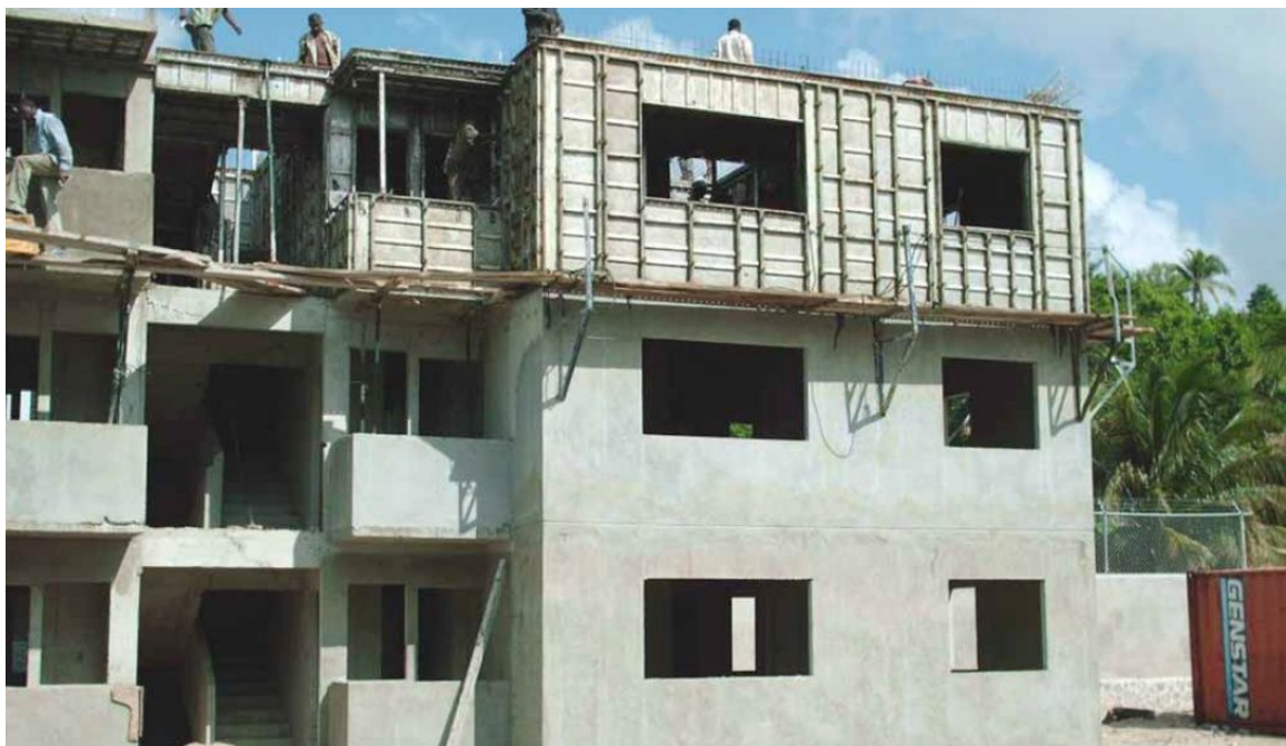
Fig 4.10 Monolithic construction cast at site( Source: DurhaInfracon- Durha Monolithic construction technology)
