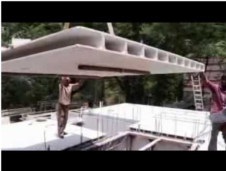
Fig 4.12 GFRG slab construction (Source: GFRG demo you tube- IITMadras)
