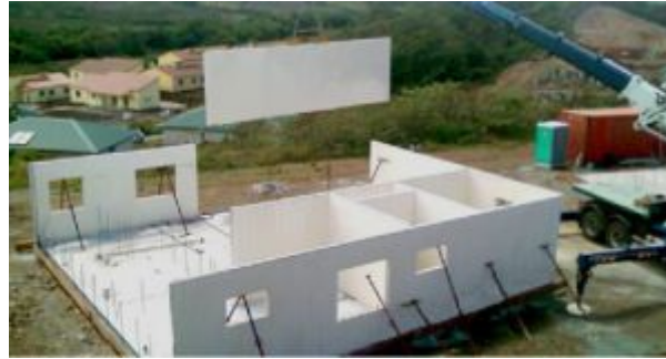
Fig 4.11 GFRG panel construction (Source: Commonfloor-Panels to replace brick walls, reduce construction time)
