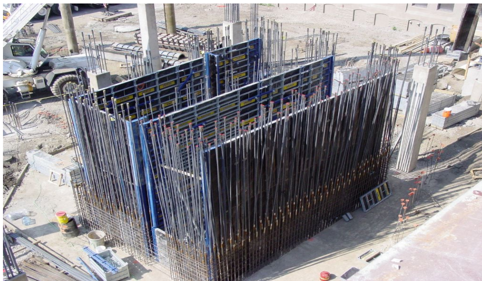
Fig 4.8 Foundation of monolithic construction (Source: Buildpedia-Concrete Reinforcing)
