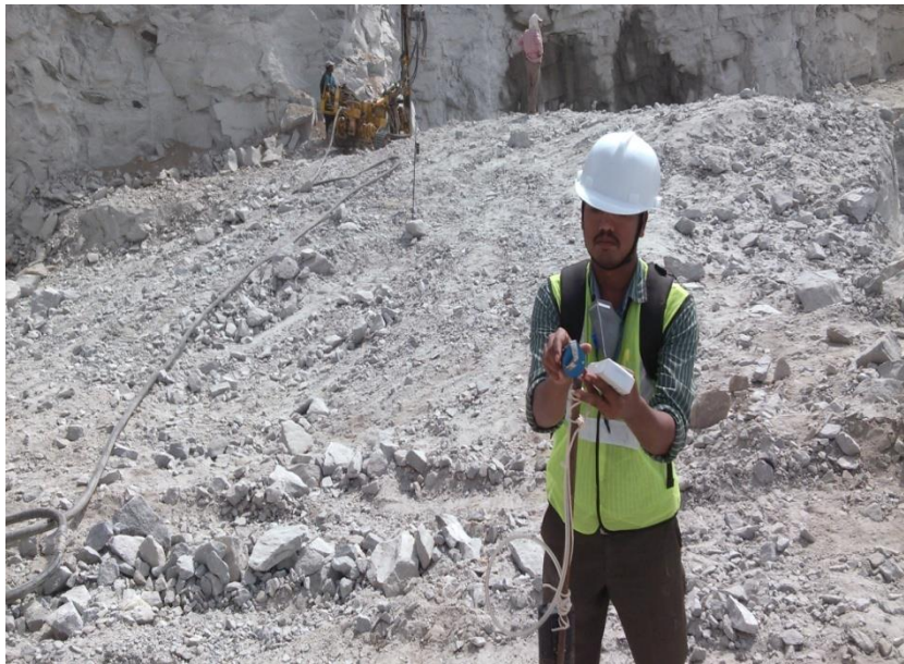
Fig. 3.24 Drilling in progress along with dust monitoring
