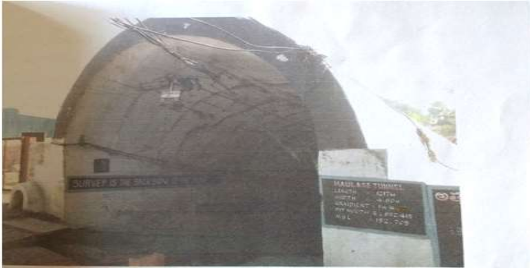
Figure 3.1 Entrance of GDK 10A incline (an underground coal mine).
