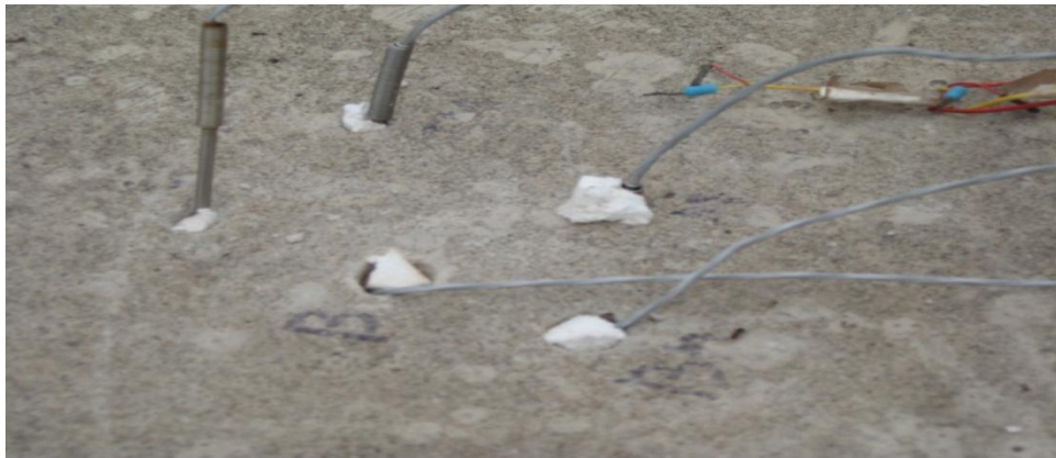
Fig 5.4 Location of drilled holes and RTD sensors
