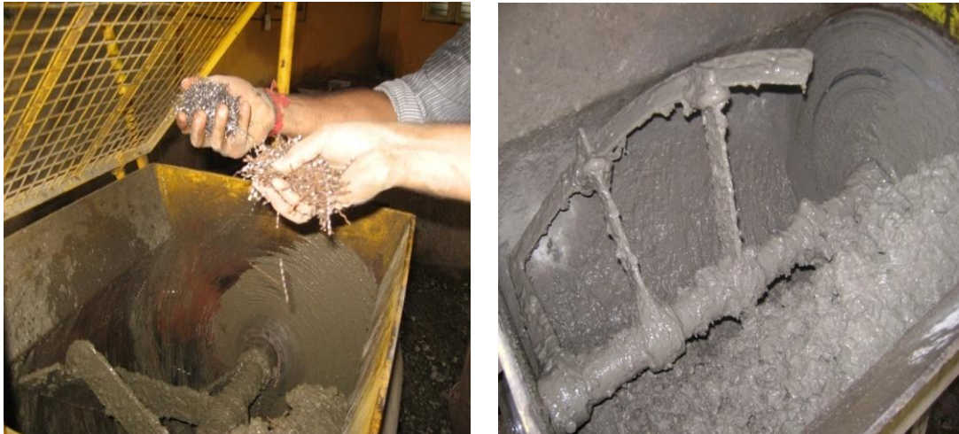
Fig. 3.2 Addition of steel fibers to the concrete and mixing of concrete in a mixer
