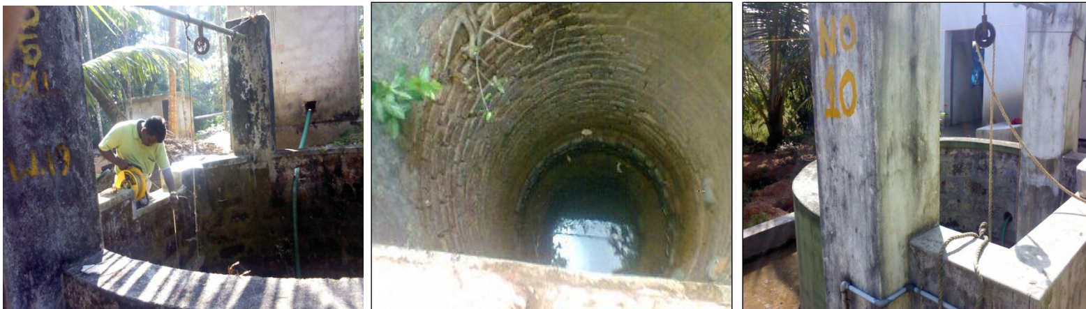
Plate: 2 Wells with Lateritic block ring and well with RCC rings
