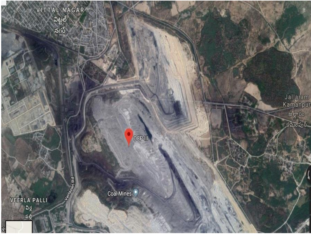
Fig. 3.13 Satellite view of Ramagundam Opencast Project-III (RGOCP-III)
