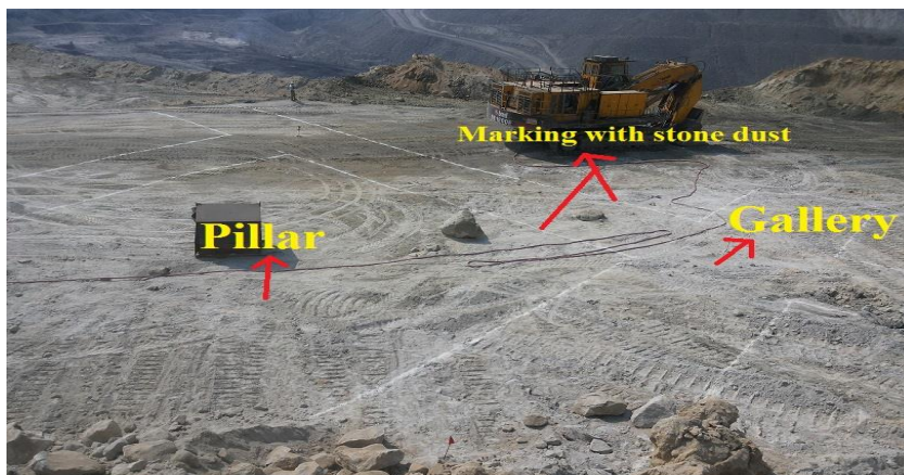
Fig. 2.3 Correlation of surface workings with old underground galleries
