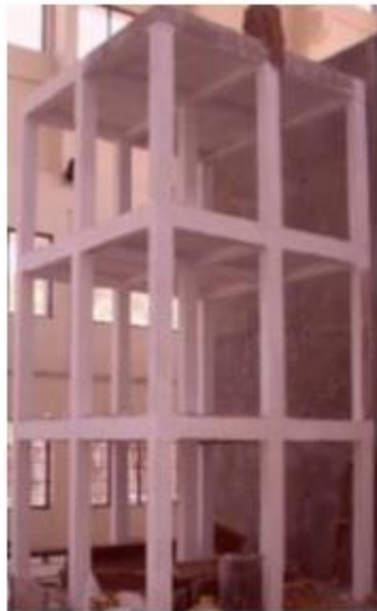
Fig. 5.1(b). Photograph of actual tested structure (photograph reprinted from Thapa M, 2009)
