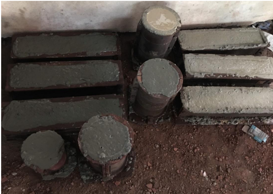
Fig. 3.6 Concrete mix casting with Waste Rock (WR)-alccofine in beams and cylinder moulds
