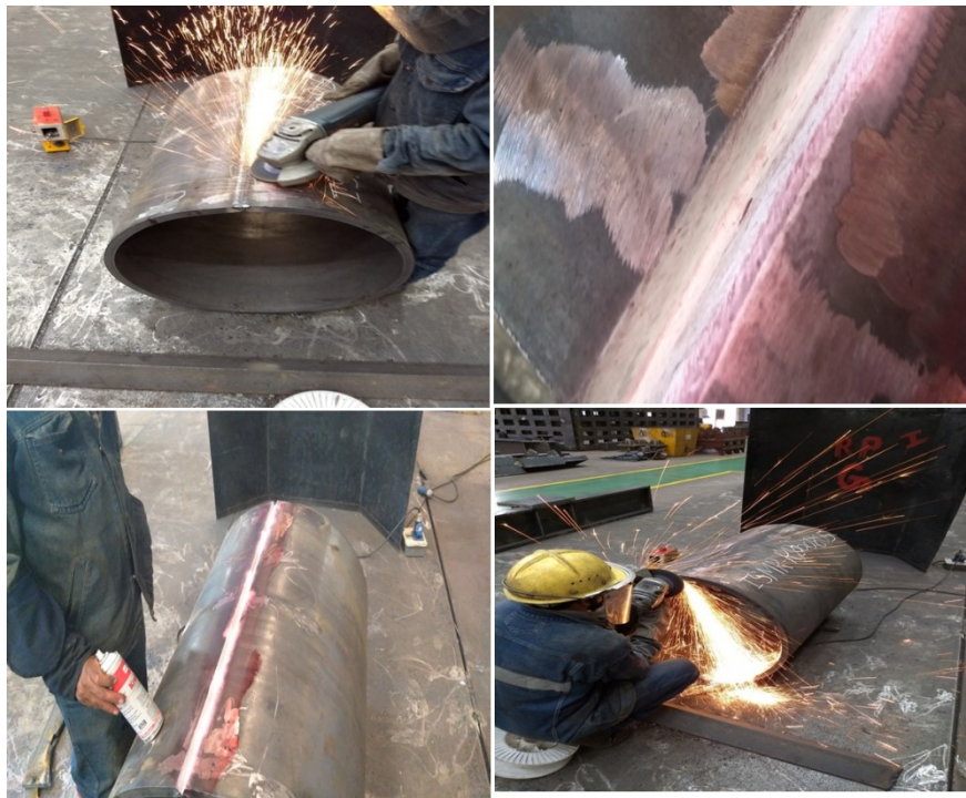
Fig. I.2 welding of classifier shell
